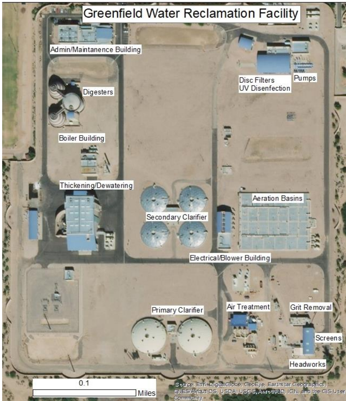
Figure 2: Aerial Photograph of Greenfield Water Reclamation Facility
